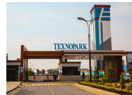
YASHNOBOD MANUFACTURING TECHNOPARK
