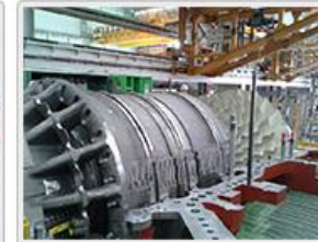
Blade Ring Dismantling, Lifting
